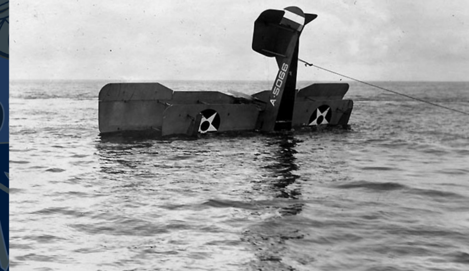
Aeromarine 40 flying boat wrecked in the Gulf of Bacabano, Cuba, 25 May 1923. This aircraft hit something on the water or broke a hole in its hull by hitting a wave, leaving the plane's wings and hull unfit for further use. It was subsequently stricken from the list of Navy aircraft
